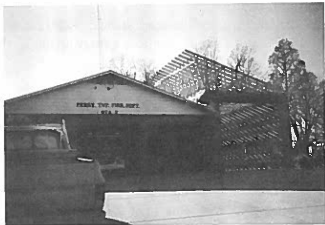
Station #2 at 11 Williams Rd under construction.
